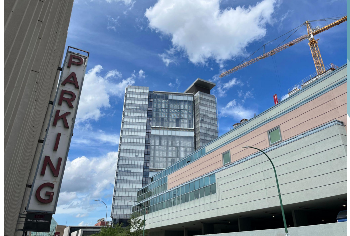
Edmonton Street Parkade Entrance
