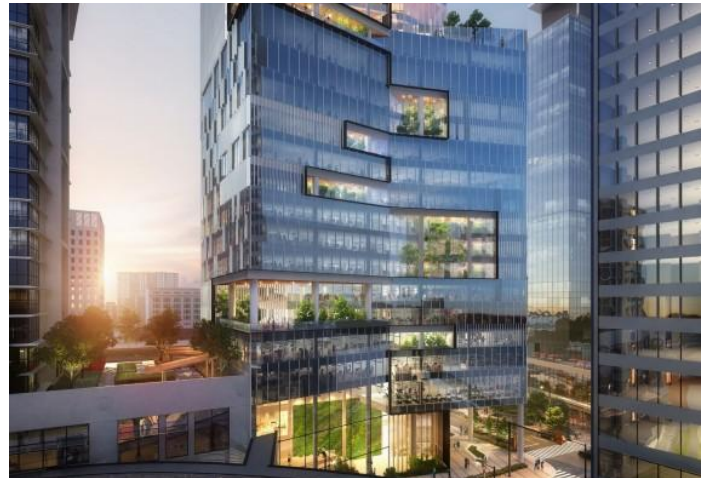
Wawanesa Headquarters (Under Construction)
